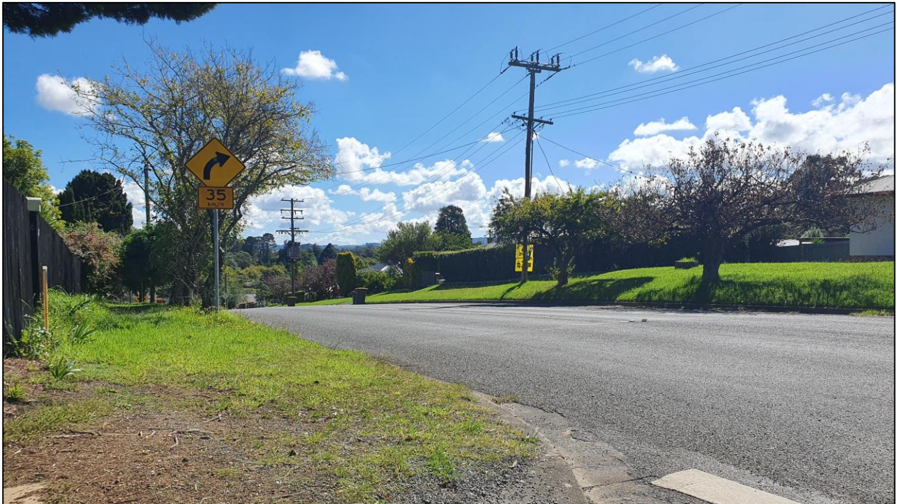
Figure 7-4 Sight distance on Darran Road looking left (north)
